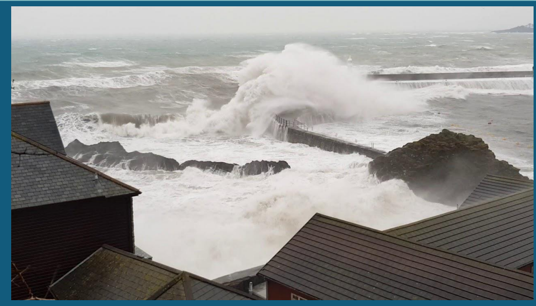
Figure 1: Overtopping at Mevagissey Harbour
